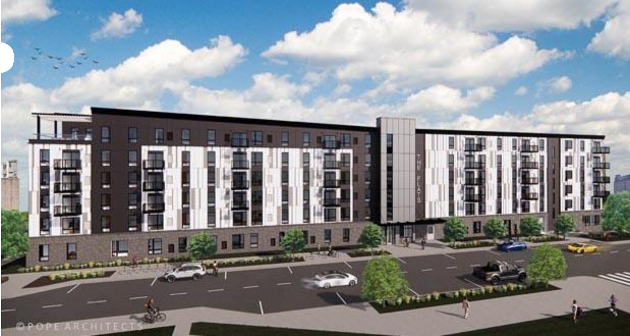
Lupe Development Partners and Wall Cos. broke ground Wednesday on The Flats at Malcolm Yards, a 143-unit affordable apartment building at 505 Malcolm Ave. in Minneapolis. (Submitted rendering: Pope Architects)
